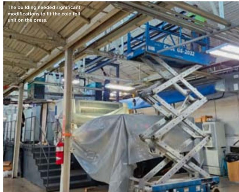
The building needed significant modifications to fit the cold foil unit on the press.
