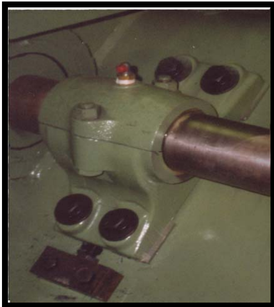
VIEW OF GLUE MECHANISM LIFT SHAFT CONVERSION
